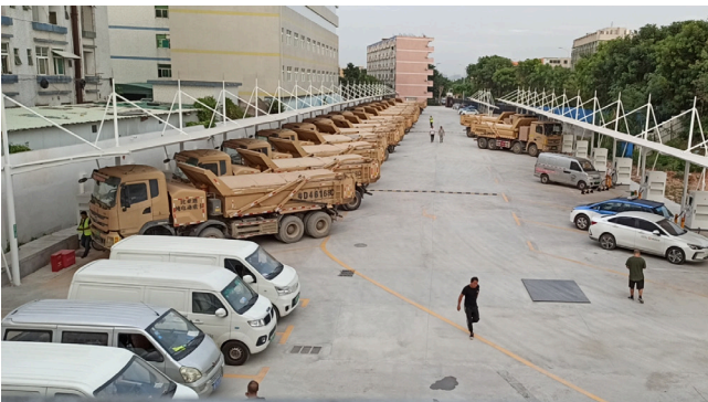
Shenzhen Longgang Truck Charging Station Fleet Charging
