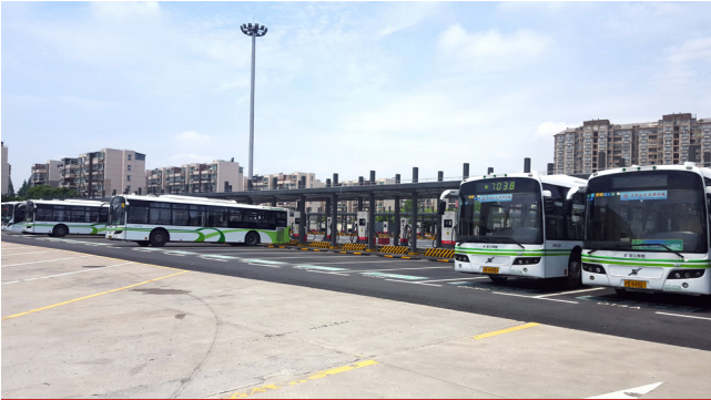
Shanghai Xinzhuang Bus Charging Station e-Bus Depot
