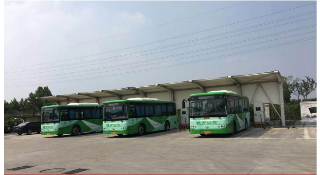
Yancheng Bus Charging Station (Stable Operation for 8 Years) e-Bus Depot
