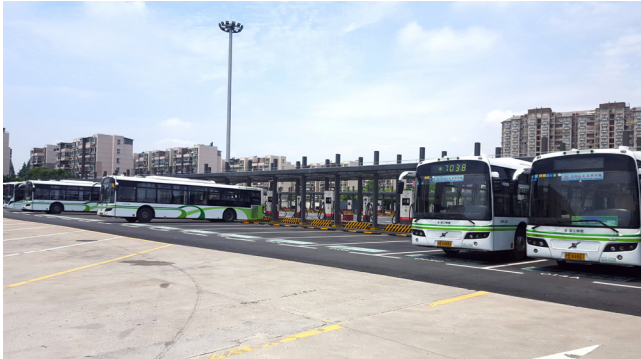
Shanghai Xinzhuang Bus Charging Station e-Bus Depot
